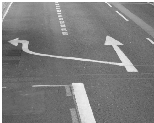
Fig. 4 Urban road traffic markings (London, Islington). Seven kinds of markings, some qualifying others. Photo: Patrick Maynard
